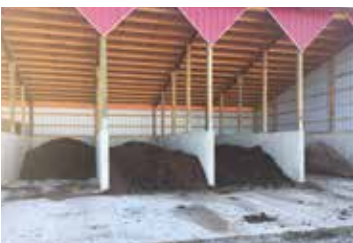
Animal mortality composting facility
