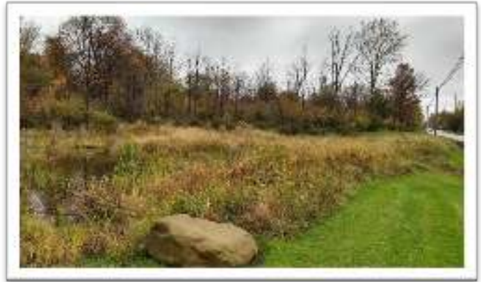
Wetland created to address excess stormwater
