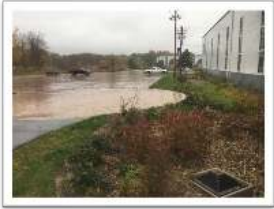
Permeable pavement with bioretention
